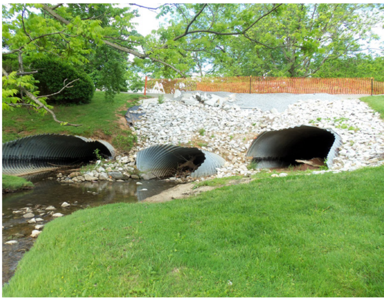
Collapsed culvert due to flooding. 186 sq. ft. flow area of clearance.
