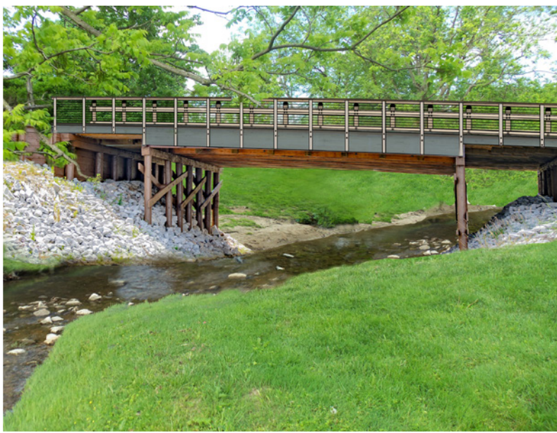
Timber bridge conceptual mock up with unrestricted water flow. 350 sq. ft flow area of clearance (47% more flow area than a culvert).
