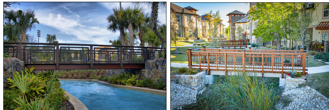
2 SHORT SPAN BRIDGE PREVIOUS WORK IMAGES NOT TO SCALE
